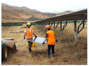
set up on 14 rows facing east and west. To increase the amount of power generated, these are designed to tilt and track the sun throughout the day. An electric motor on each row operates the tilting, guided by a geo-spatial timer. There is also a fixed (non-tilting) set of panels that faces north.
