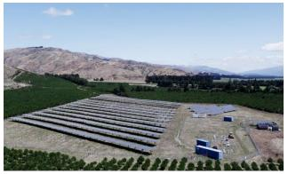
panels automatically tilt to follow the sun throughout the day, and it generates power from light reflecting up from the ground and on to the bi-facial panels, as well as down from the sun.
